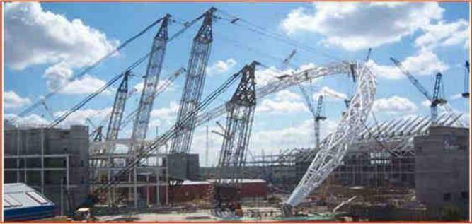
Fig 4. Turning Mast
