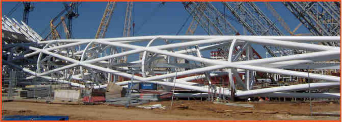
Fig 3. Segment of Truss
