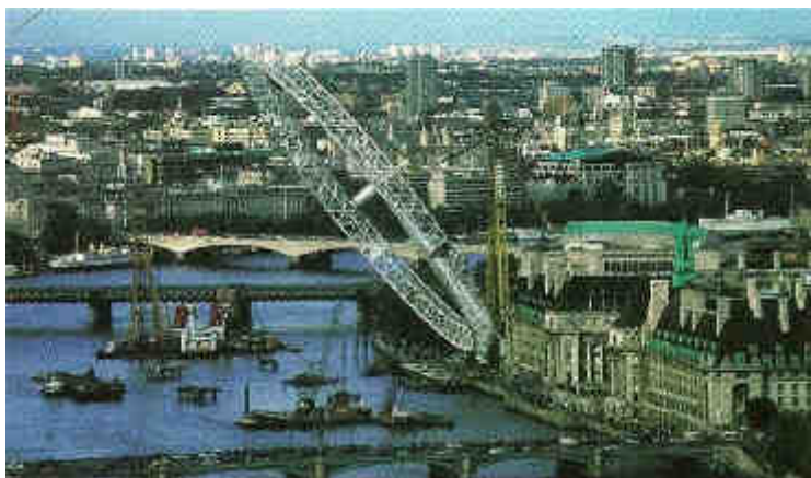
Fig 18. London Eye - raising the wheel (© Nick Wood)
